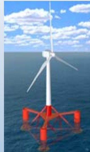
Wind Turbine on Dutch Tri-floater
